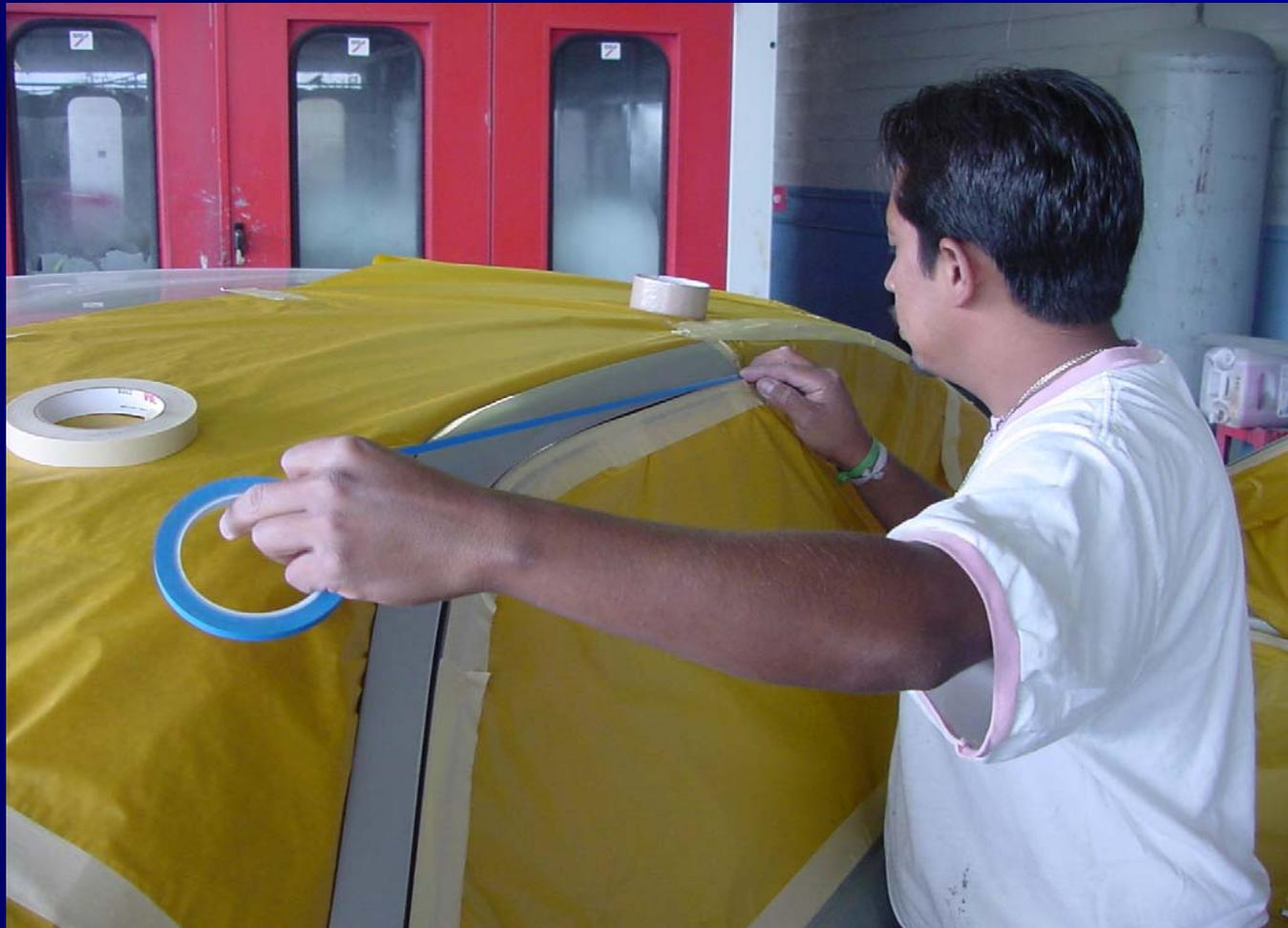
Technician is applying a final layer of tape to the door window molding.
